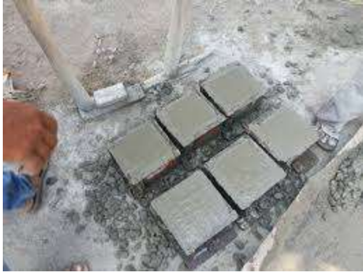
casting of cubes
